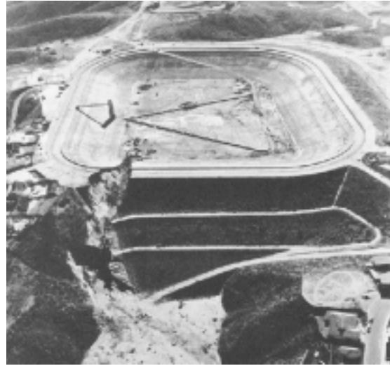
Figure 1: Piping failure at Baldwin Hills Reservoir, California 1963 (Cedergren, 1967)
